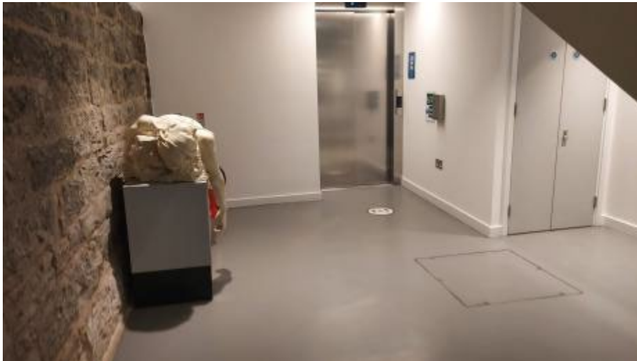
The space between the lift and the corridor with the toilets.
