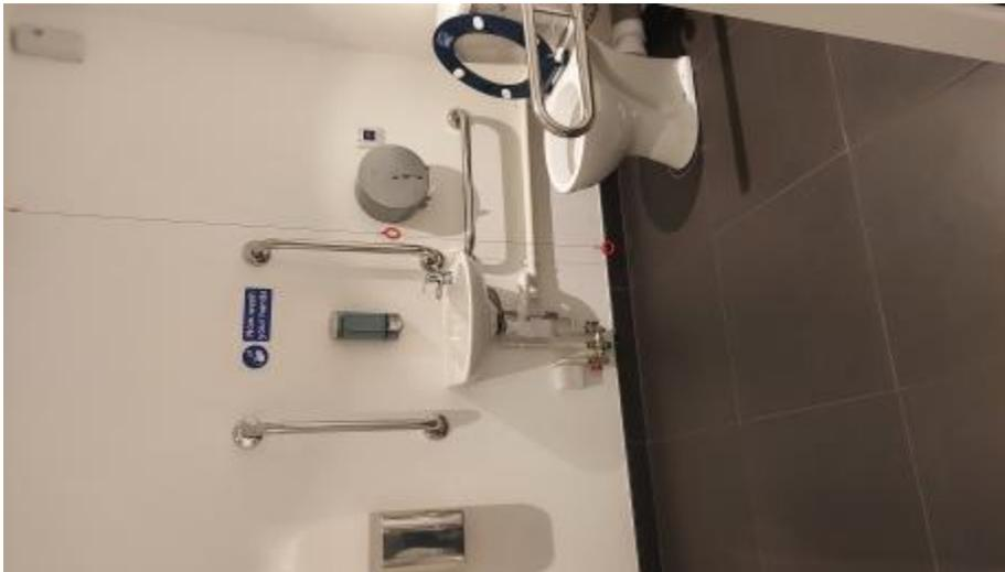
The accessible toilet. Showing the handrails, lowered sink and hand dryer and pull cord.
